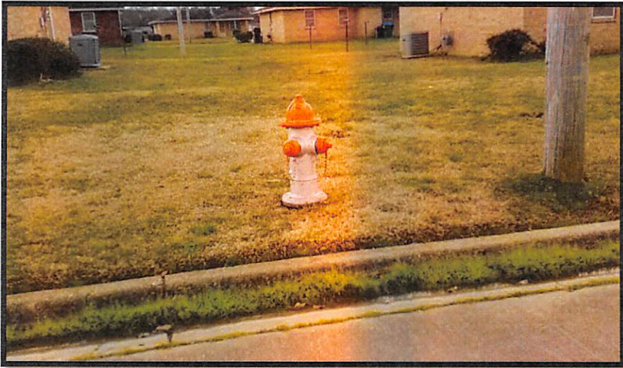
Hydrant and water main access point on southwestern corner of central area.
